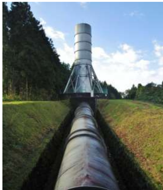
Figure 5.22: A balance chimney
